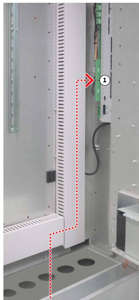
b) Cable entry from bottom
